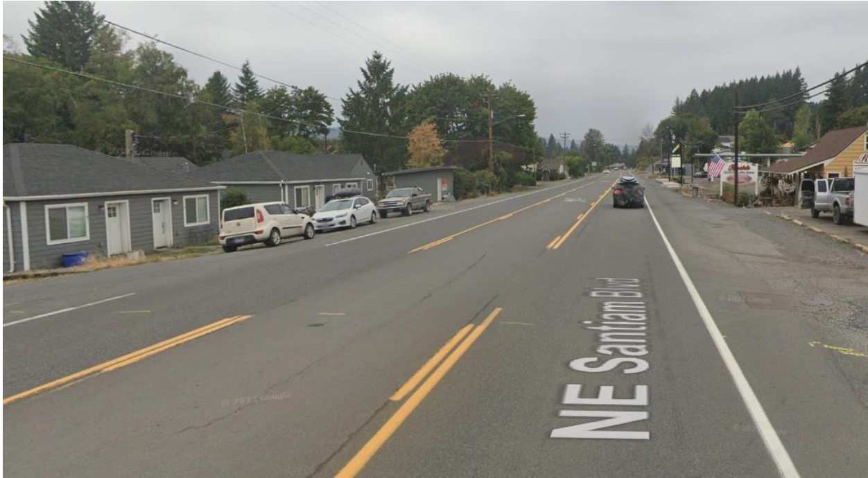
Figure 4-3. OR 22/NE Santiam Boulevard at NE 7th Avenue Facing West. There are no sidewalks, and residential and commercial uses are adjacent to the right-of-way.
