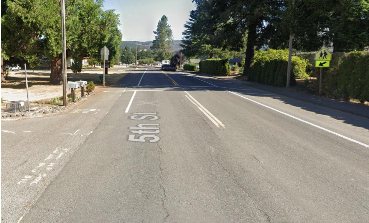
Figure 3-2. OR 226/5th Street at the Mari-Linn School Facing North. No bike lanes or enhanced crossings exist, and there is only a narrow sidewalk on one side.
