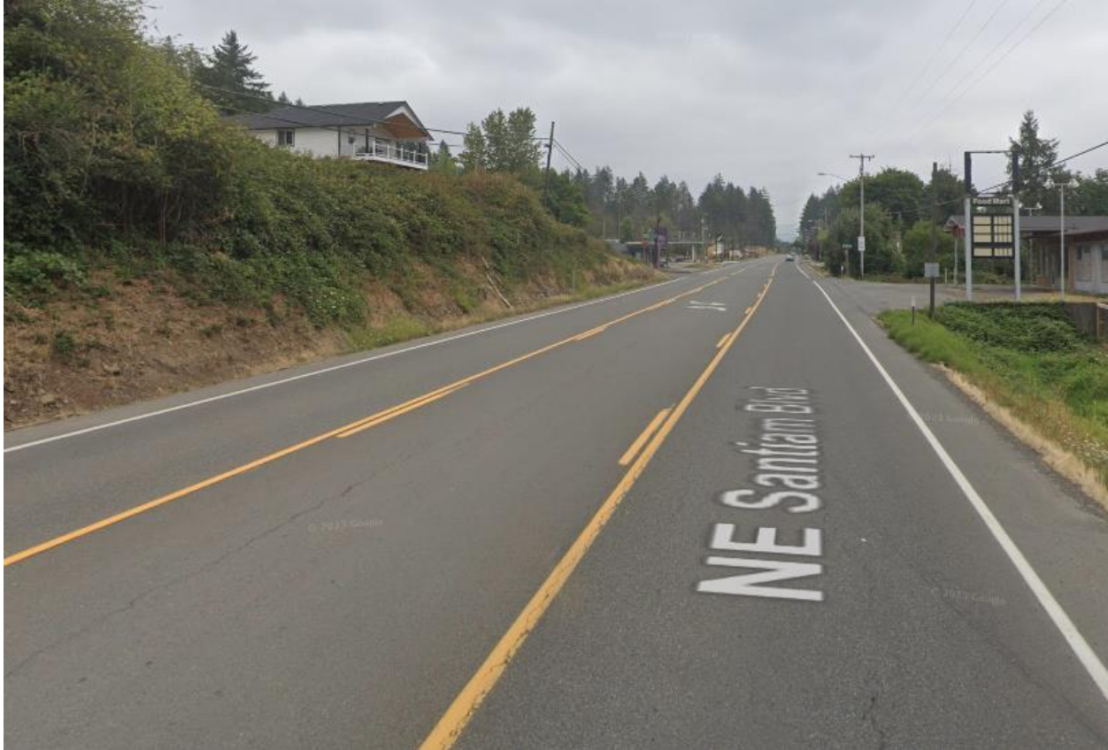
Figure 4-2. OR 22/NE Santiam Boulevard at NE 3rd Avenue facing east. There are no sidewalks, and narrow shoulders are present.
