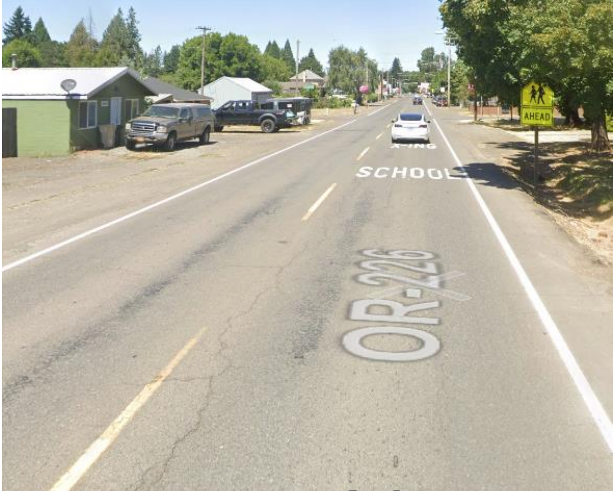
Figure 2-2. OR 226/S Main Street in Scio Looking North from SW 5th Avenue. No sidewalks, bicycle lanes, or marked crosswalks are present on this segment.
