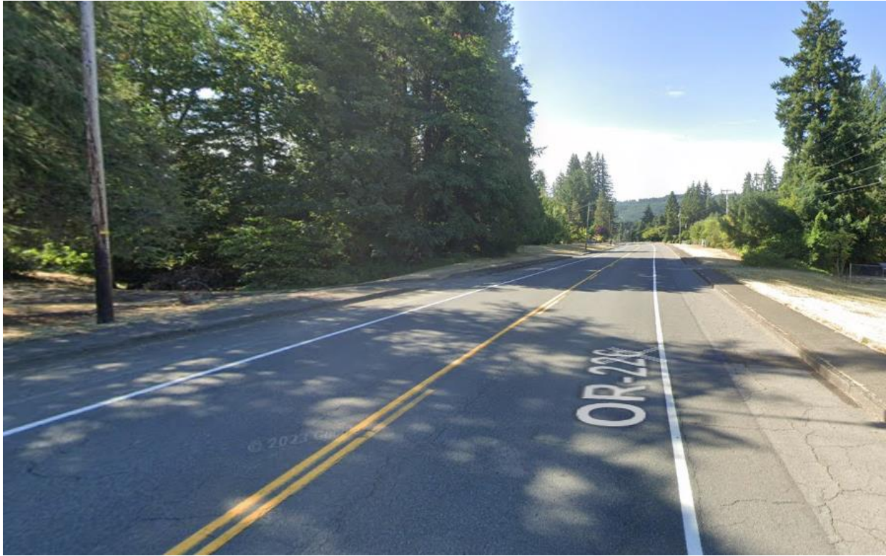
Figure 3-3. OR 226 Facing South. Wide shoulder and sidewalks are present, but there are no bicycle facilities
